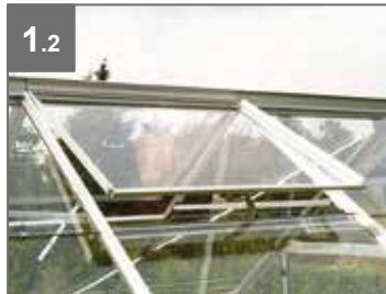
1.2 Window Exterior view
